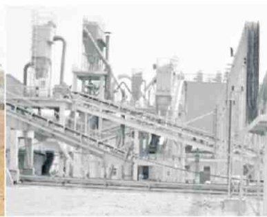
A Cement Factory
